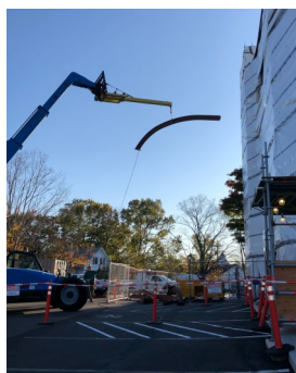
The pieces making up the steel supporting structure were delivered on November 5 and lifted one by one.
